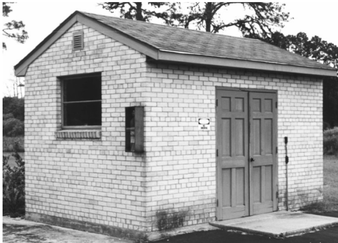
Figure 78. Buildings at Welaka National Fish Hatchery, Florida. Upper: Service Building or Combination Office-Three Bay Garage. Center: Fertilizer House. Bottom: Oil and Paint House.. These buildings were constructed in 1959 and are virtually identical to their counterparts at McKinney Lake National Fish Hatchery. The only difference is material, brick at Welaka and concrete block at McKinney Lake [Source: Kanaski 2001].
