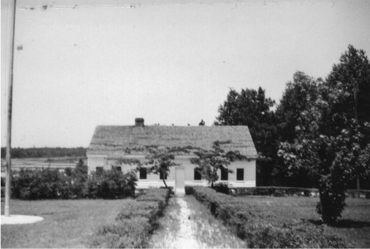
Figure 57. "Old" Office-Shop-Garage, front elevation, ca. 1947 [Source: D. C. Booth Historic National Fish Hatchery and Archives].
