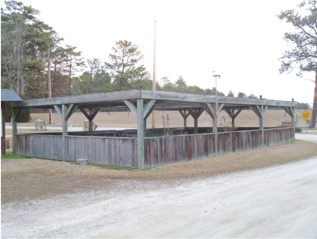
Figure 37. Covered Observation Ponds, southwest corner, 2014 [Bradford 2014].
