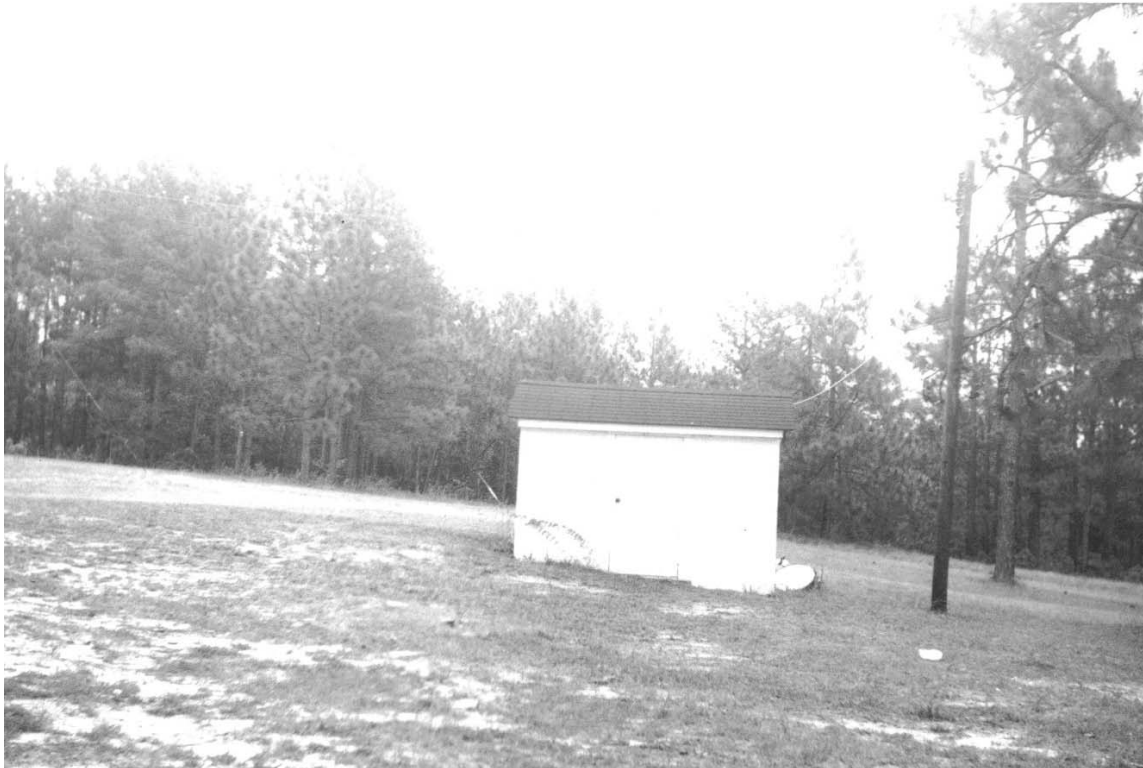
Figure 56. Pump House, which located between Quarters 1 and Quarters 2, ca. 1971 [Source: D. C. Booth Historic National Fish Hatchery and Archives].
