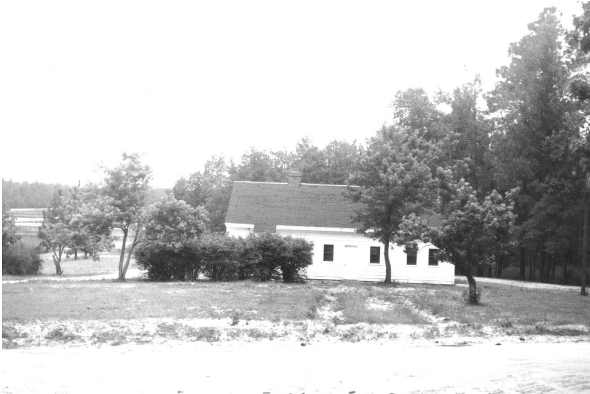
Figure 59. "Old" Office-Shop-Garage, front elevation, ca. 1954. Note the shrubs that once flanked the sidewalk are gone [[Source: D. C. Booth Historic National Fish Hatchery and Archives].
