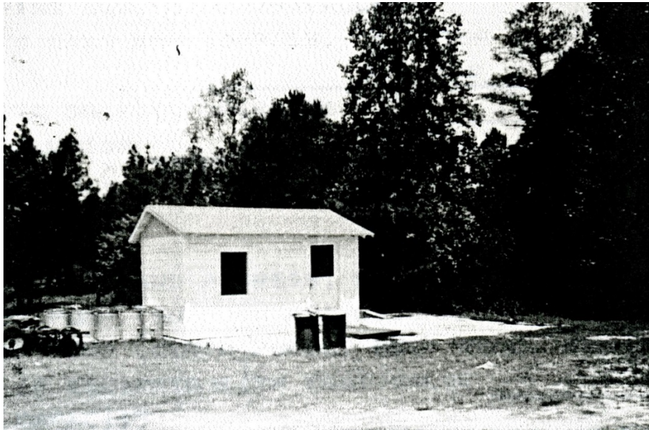
Figure 62. Temporary Oil House, southeast corner, ca. 1947 [Source: D. C. Booth Historic National Fish Hatchery and Archives].
