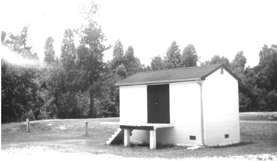
Figure 32. Fertilizer House, northeast corner, ca. 1971 [Source: D. C. Booth Historic National Fish Hatchery and Archives].
