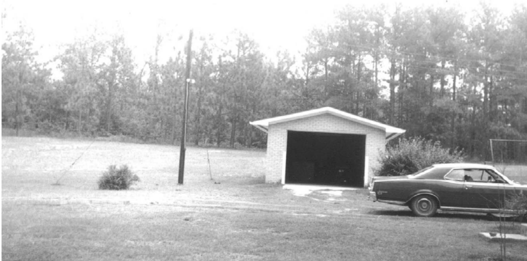
Figure 54. Detached brick one-car garage, front elevation, ca. 1971 [Source: D. C. Booth Historic National Fish Hatchery and Archives].
