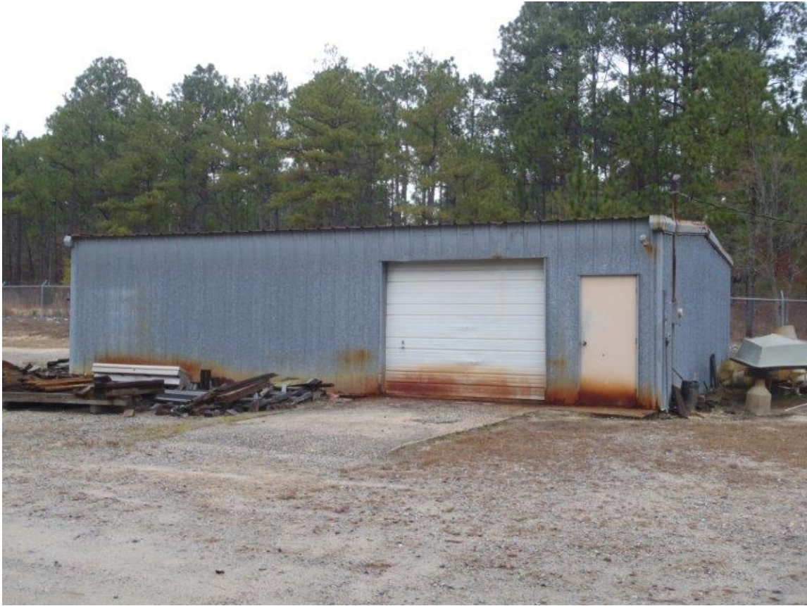
Figure 65. Metal Storage Building, 2013 [Bradford 2013].
