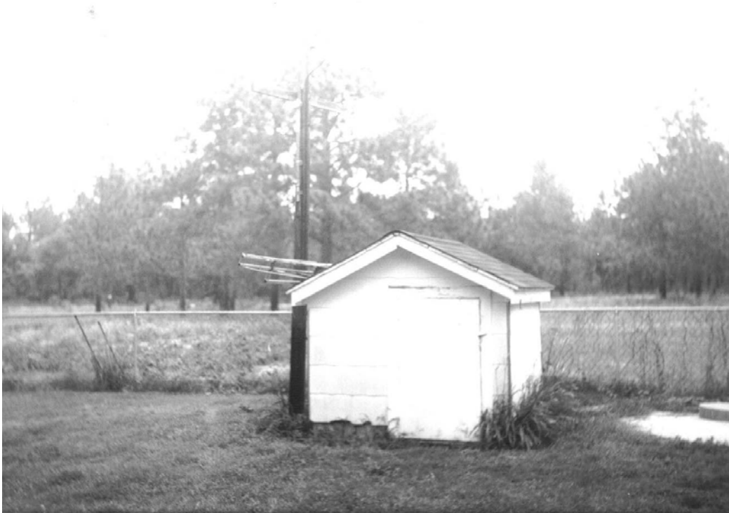
Figure 74. Pump House, ca. 1971 [Source: D. C. Booth Historic National Fish Hatchery and Archives].
