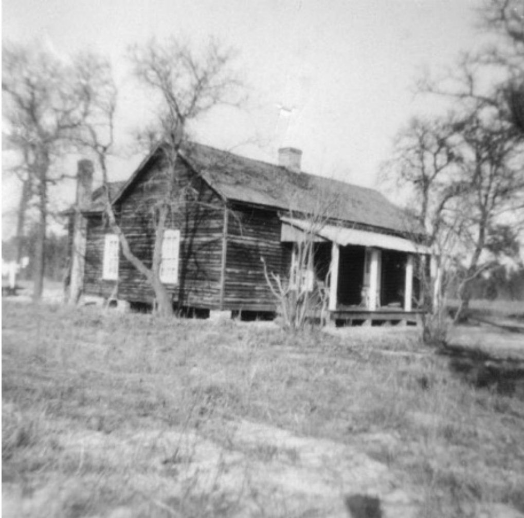
Figure 70. The original look of Quarters 3, ca. 1949 [Source: D. C. Booth Historic National Fish Hatchery and Archives].
