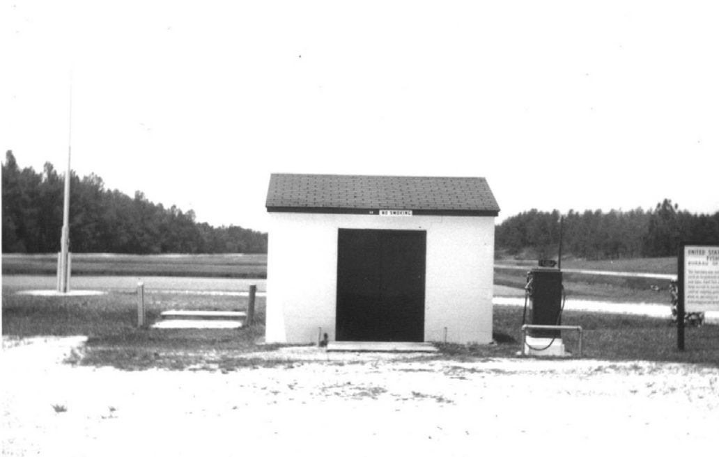
Figure 34. Oil and Paint House, front elevation, ca. 1971 [Source: D. C. Booth Historic National Fish Hatchery and Archives].
