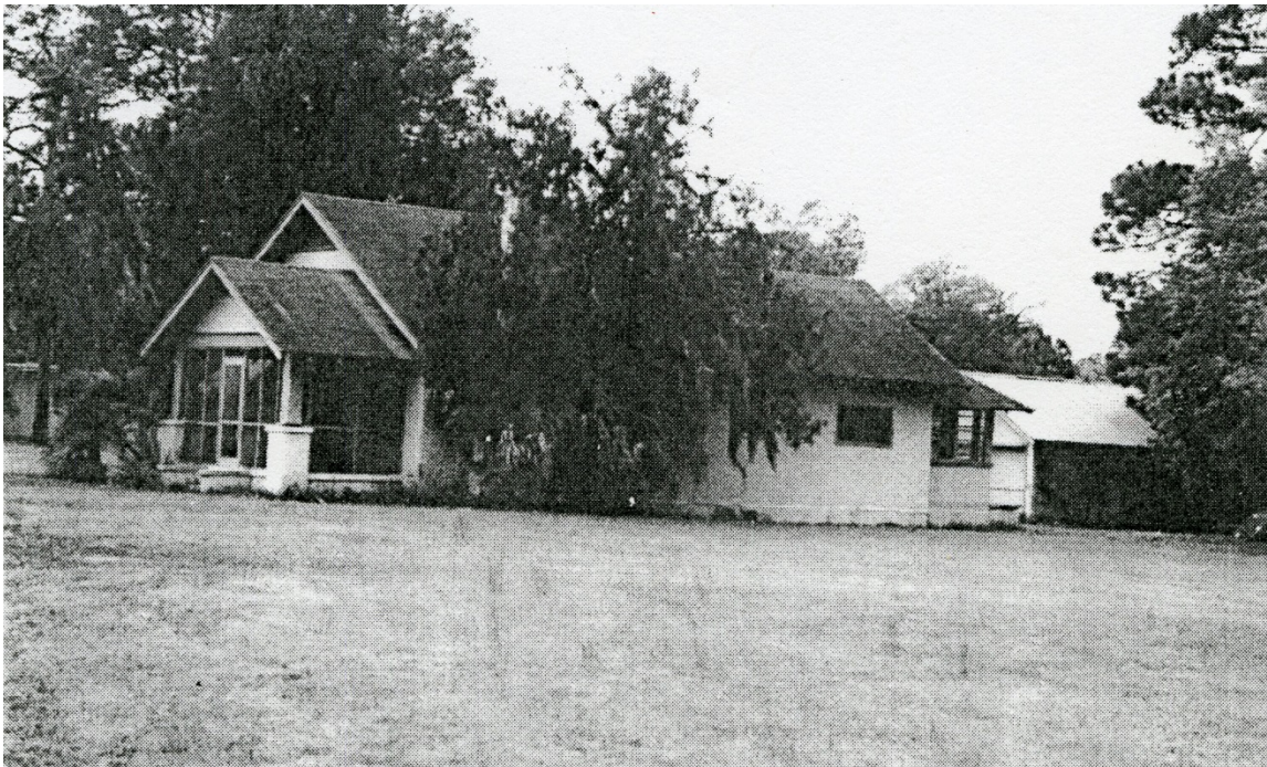
Figure 83. One of the bungalows built for the state hatchery at Welaka, Florida, ca. 1927. The state hatchery and game farm was purchased by the Resettlement Administration about the same time. The hatchery was transferred to the Bureau of Fisheries in 1938. The hatchery was renamed Welaka National Fish Hatchery [Source: Kanaski 2001].
