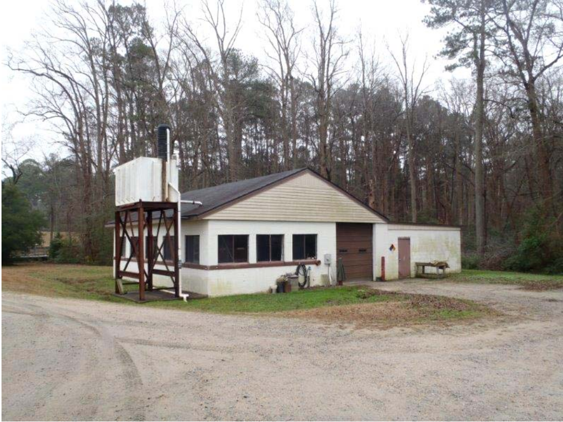
Figure 30. “New” Holding House, 2013. Note the concrete block addition with shed roof [Bradford 2013].
