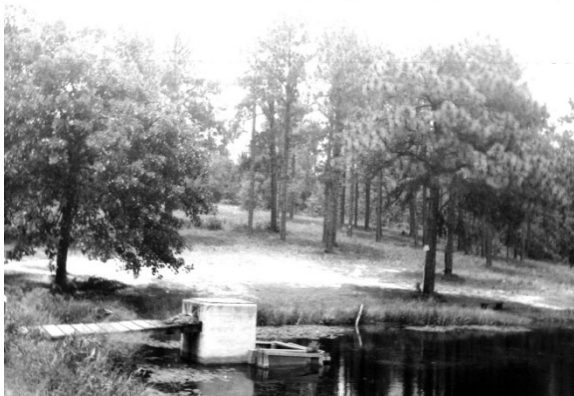
Outlet box or drain.
