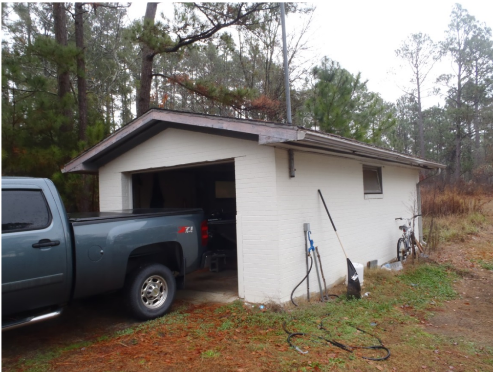
Figure 47. Quarters 1's detached one-car garage, southwest corner, 2013 [Bradford 2013].
