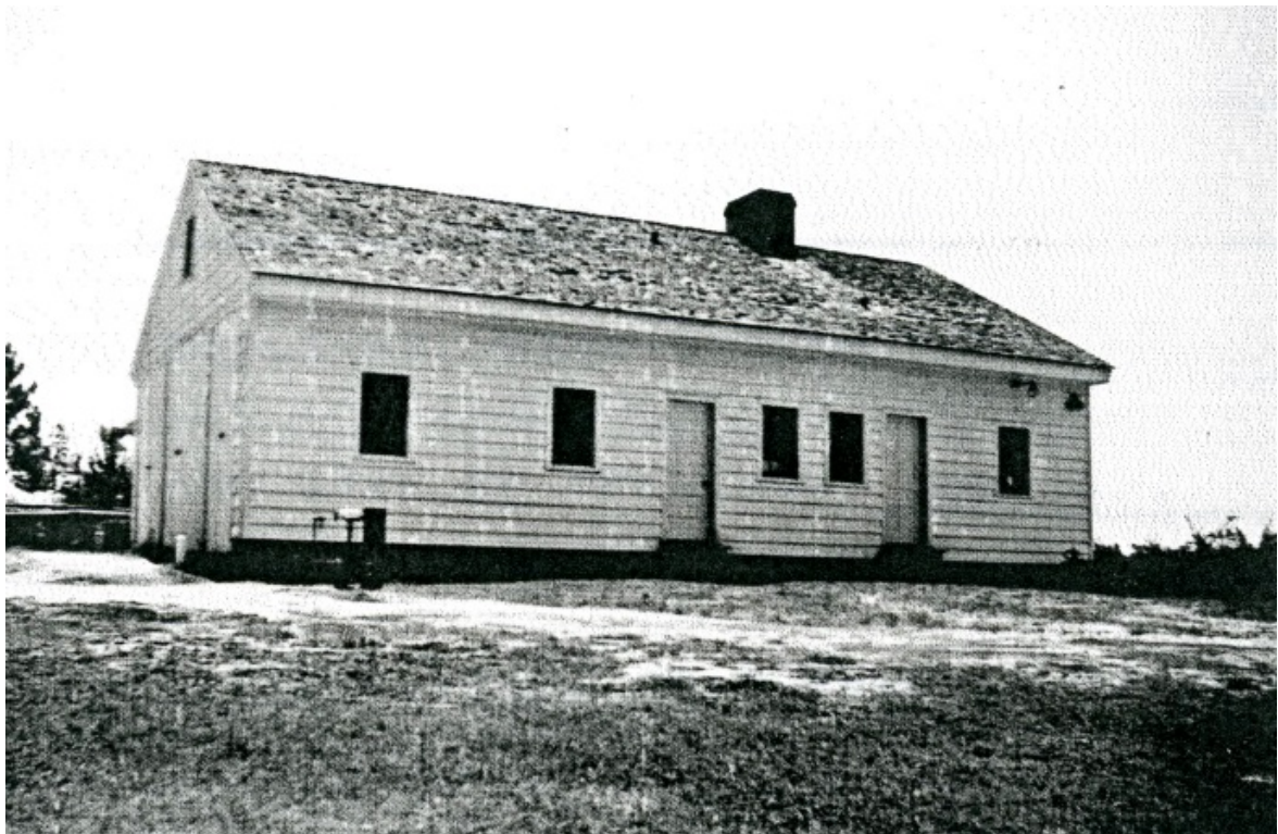
Figure 60. "Old" Office-Shop-Garage, rear elevation, ca. 1947. The doors lead into the shop and the rear office [Source: D. C. Booth Historic National Fish Hatchery and Archives].
