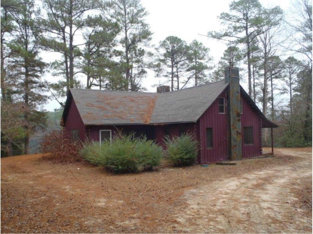
Figure 67. Lodge and Meeting Rooms, 2013 [Bradford 2013].
