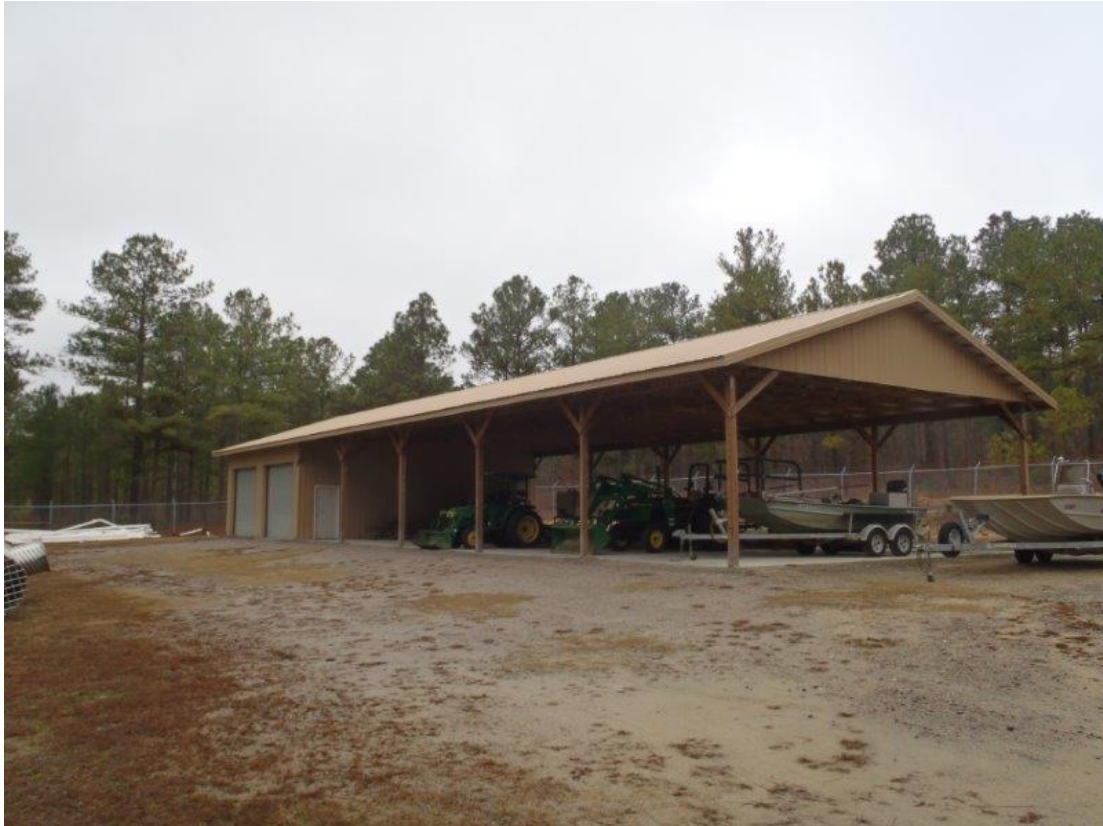
Figure 64. Replacement Pole Shed, 2013 [Bradford 2013].
