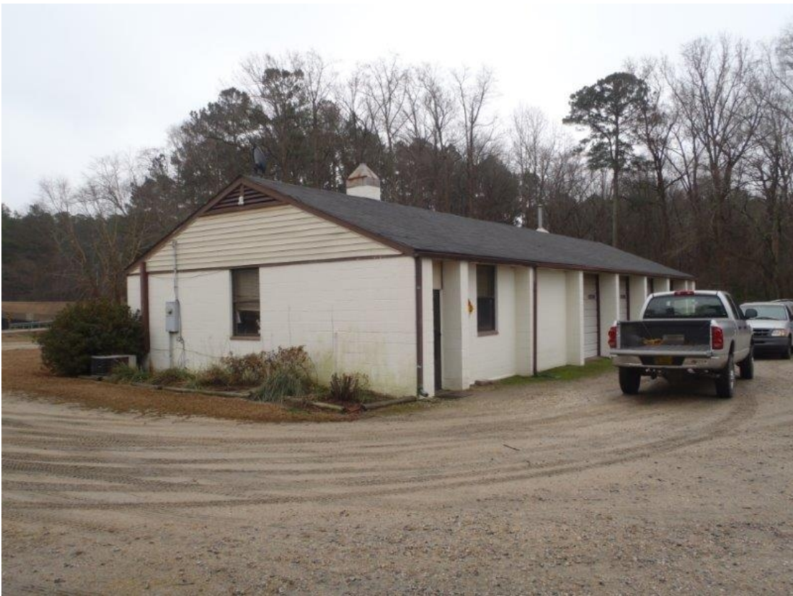
Figure 26. "New" Service Building, northwest corner, 2013 [Bradford 2013].
